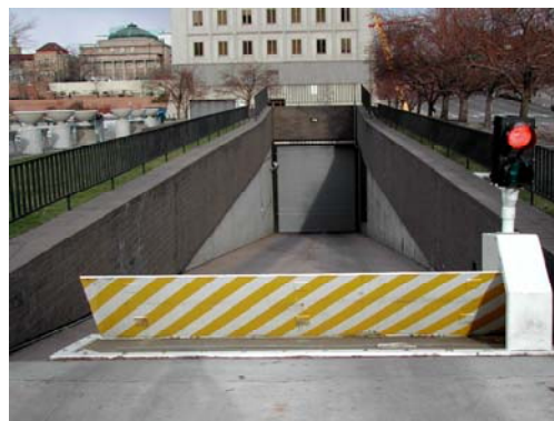
Vehicle barriers such as this and other access control measures assist in managing vehicles approaching a submerged access point.
